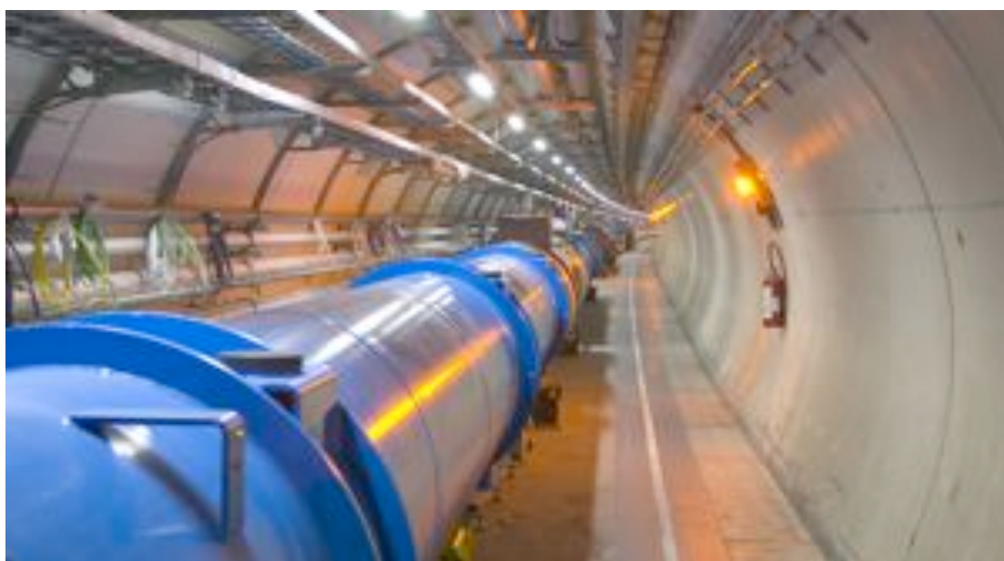
Figure 1. The LHC tunnel
