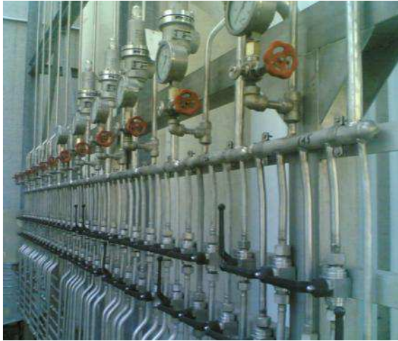
Figure 8.39: “manual” control panel of the high pressure storage (left) and high pressure vessels (right)
