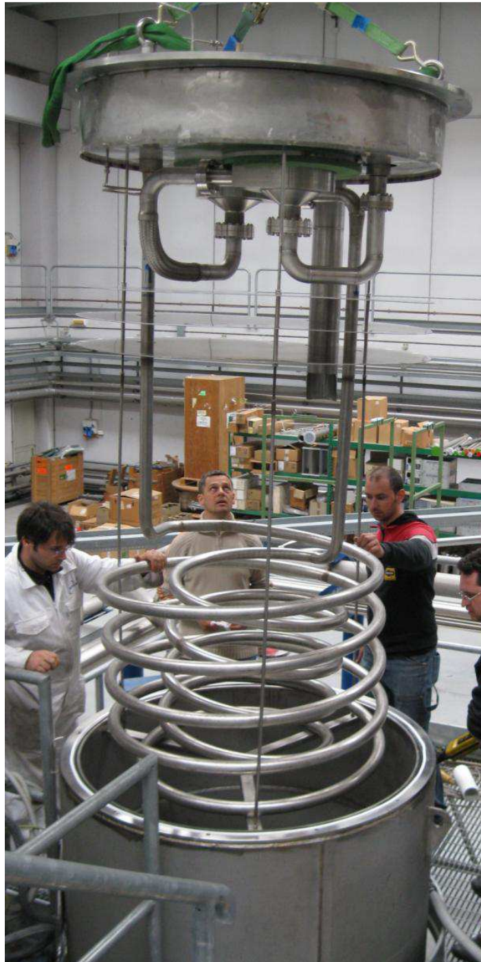
Figure 8.47: installation of the heat exchanger in the Auxiliary Cold Box
