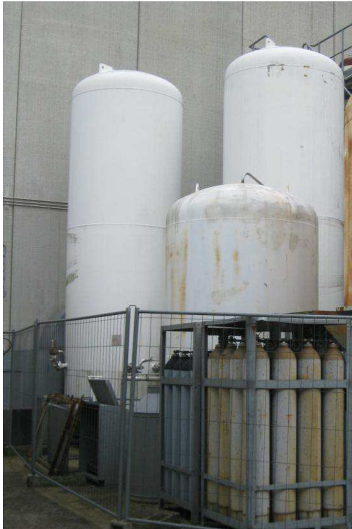
Figure 8.38: present buffer system for pure helium gas at INFN-LNL
